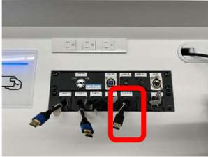
2. Connect one of the cables from [HDMI1], [HDMI2], [USB-C1], or [USB-C2] on the operation desk to the brought-in PC.
